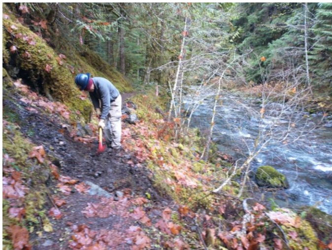
Dirt work done.
