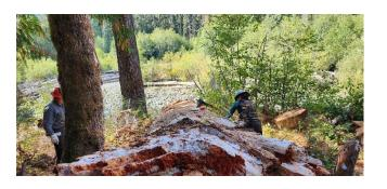
We sawed out a 50" rotten snag that had fallen at the downriver end of the realignment. Easy to cut due to being so rotten, but we had to dig a lot underneath it to keep the saw chain out of the dirt. Thus all the sawdust covering the back of my vest.
