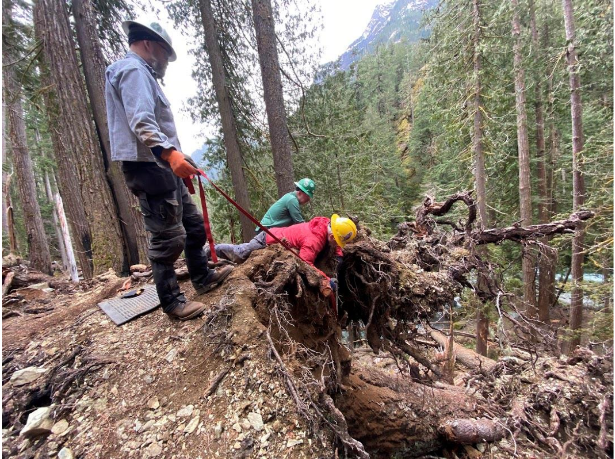
FEEDING THE STRAP UNDER THE ROOT.
