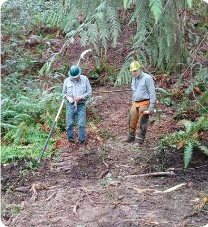
Tom Mix and Jim Hollatz planning a culvert installation.
