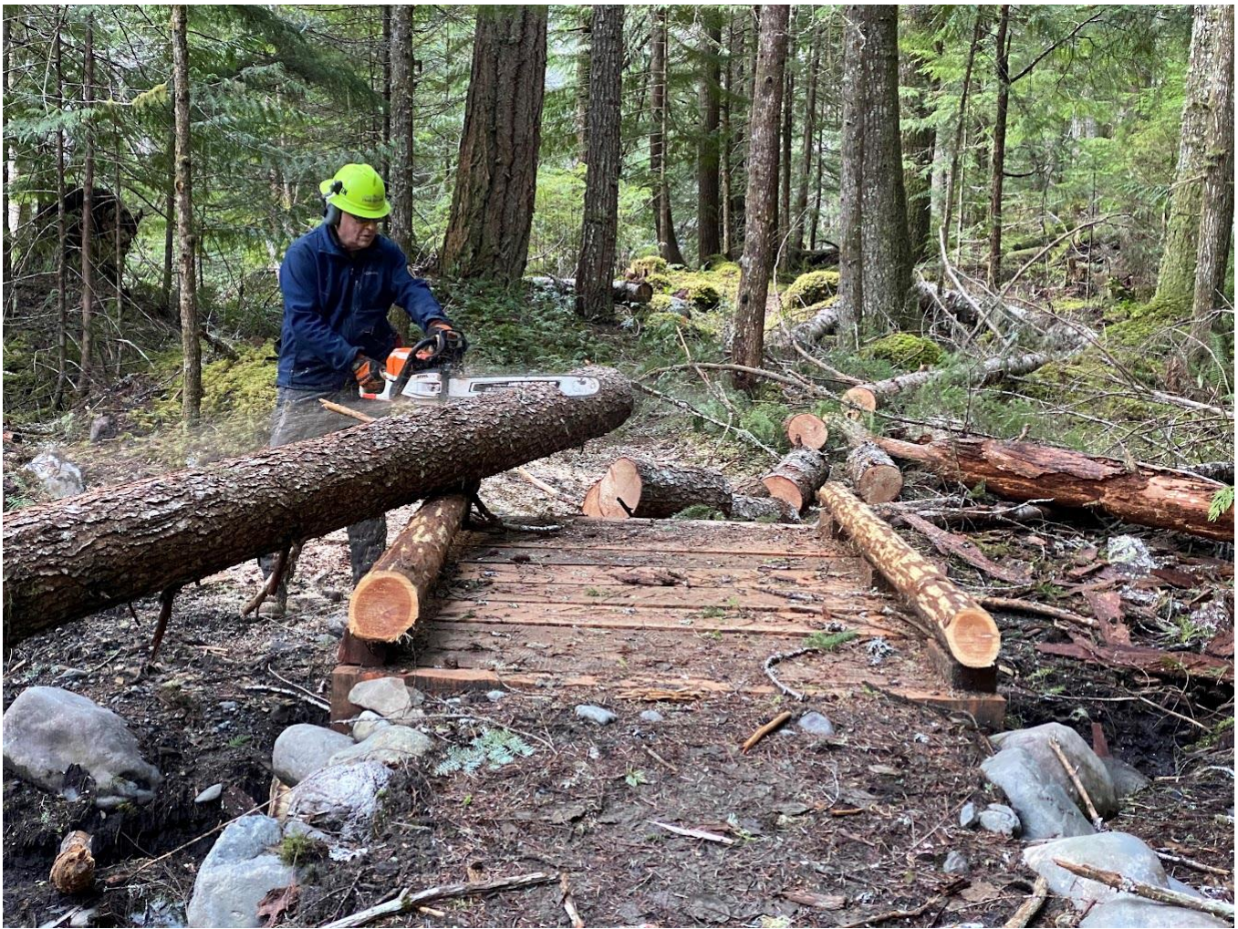
This tree landed squarely on the brand-new puncheon just built last August (teamwork between GWTC and WTA). Fortunately, the new bullrails are larger than normal, fresh and new, so they protected the puncheon. No damage!
