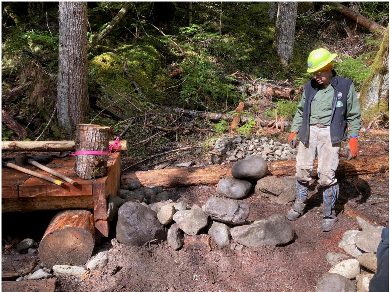
Progress happening on the rock ramp for the upstream side of the puncheon built last August. By the end of the day this was a lot higher! We have exhausted our supply of rock at the job site so the team is having to search elsewhere and transport the rock. Super time consuming.
