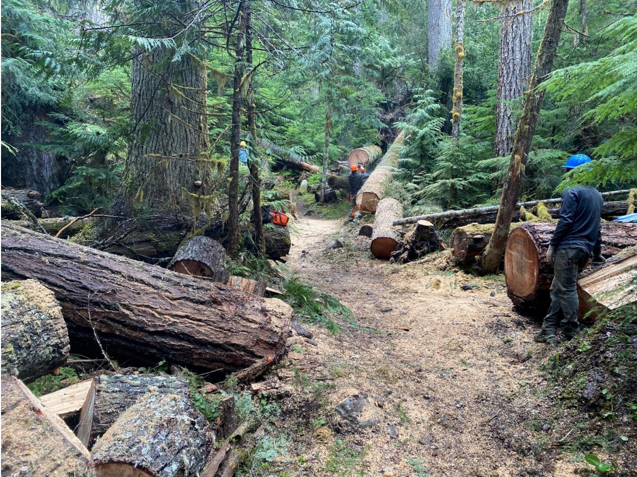
FINISHING TOUCHES – ANGLING THE LOGS TO THE LAY OF THE TRAIL.
