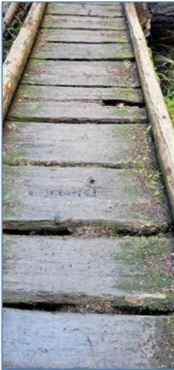
This is the bridge that crews will be replacing.
