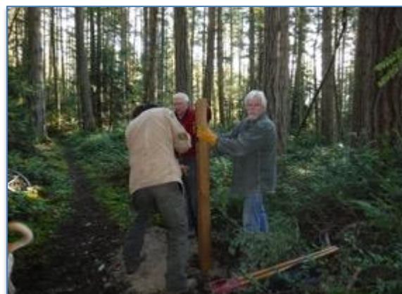
Installation of an intersection sign.
